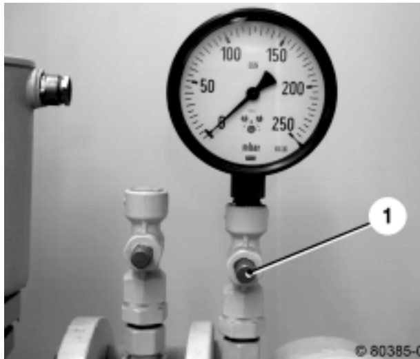
A 1 Pressure gauge gas regulating line
